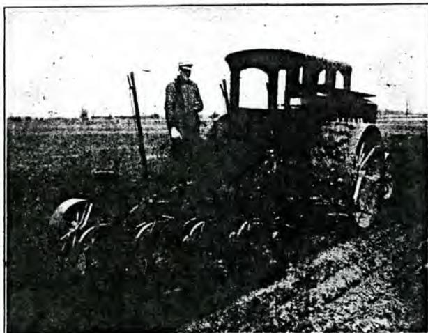
Rating 30 h. p.; 20 d. b.; 30 b. h. p.; 2 cyl.; 4 wheels; 2 drivers; speed  $1\frac{1}{2}$  to 3; 500 r. p. m.; pulley 18x8; front wheel 38x8; drivers 60x18; tanks, gasoline 3, kero. 16; cooling system, radiator; weight 8,000; price \$1,650.
