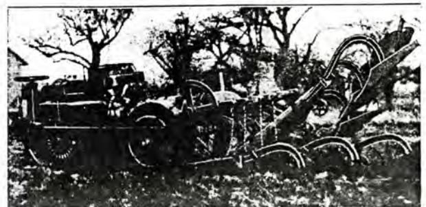
Rating 34 h. p.; 27 d. b.; 30 b. h. p.; 4 cyl.; 1 wheel and 2 drums; 2 drivers; speed  $1\frac{1}{2}$  to 8; diam. pulley 6 in.; face front wheel 14; drums 36x24; length 140; width 74; height 58; weight 4,500; furnished with or without plows (3-bottom, two-way); orchard cultivators; wagon bed; dump box; drum covers for rolling; Continental motor. Will be ready for fall trade.
