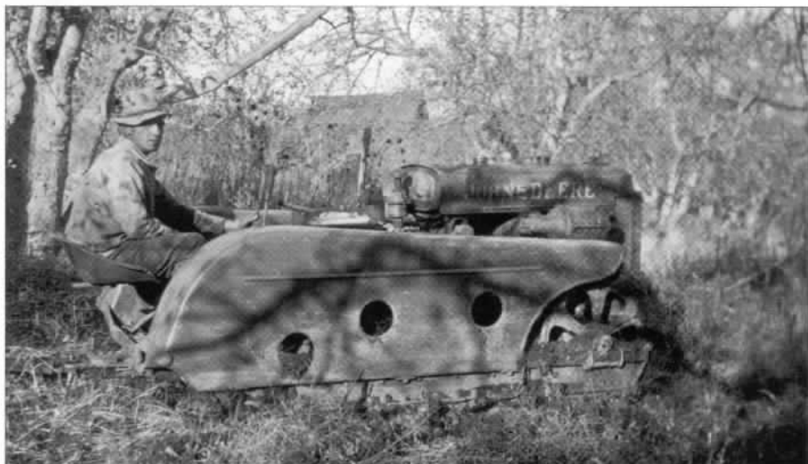
Left: The Lindeman-John Deere "GPO" Crawlers (usually just referred to as the "GPO" Crawler) were originally fitted with fenders. However, those run in more open terrain typically had the fenders removed, thus making service more accessible. As of this time, most of the fenders have been lost.
