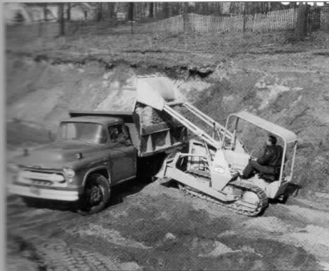
Here: With the combination of a Maine Steel 4DC Bulldozer, a Main Overhead Shovel with 3/3-cubic-yard capacity, and a "420" Crawler with five-roller tracks and an industrial yellow paint job, it was no trick at all to move a lot of dirt in a short time. The street shoes limited dirt work to reasonably dry conditions.
