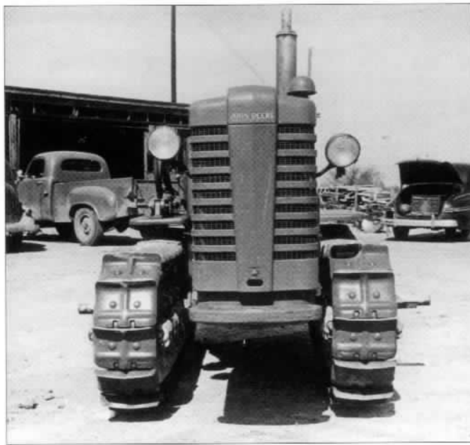
Top: Within a year after acquiring the Yakima Works, there had been improvements made to the crawler attachment for the Model "M", and the John Deere Dubuque Tractor Works was creating its own experimental crawlers with the designation "XMC". Shown here is "XMCOR", the first of them, with a five-foot scraper. Note the data recorder (round device) on the right side near the dash. Bottonfield Ranch; Laredo, Texas. March 1948.
