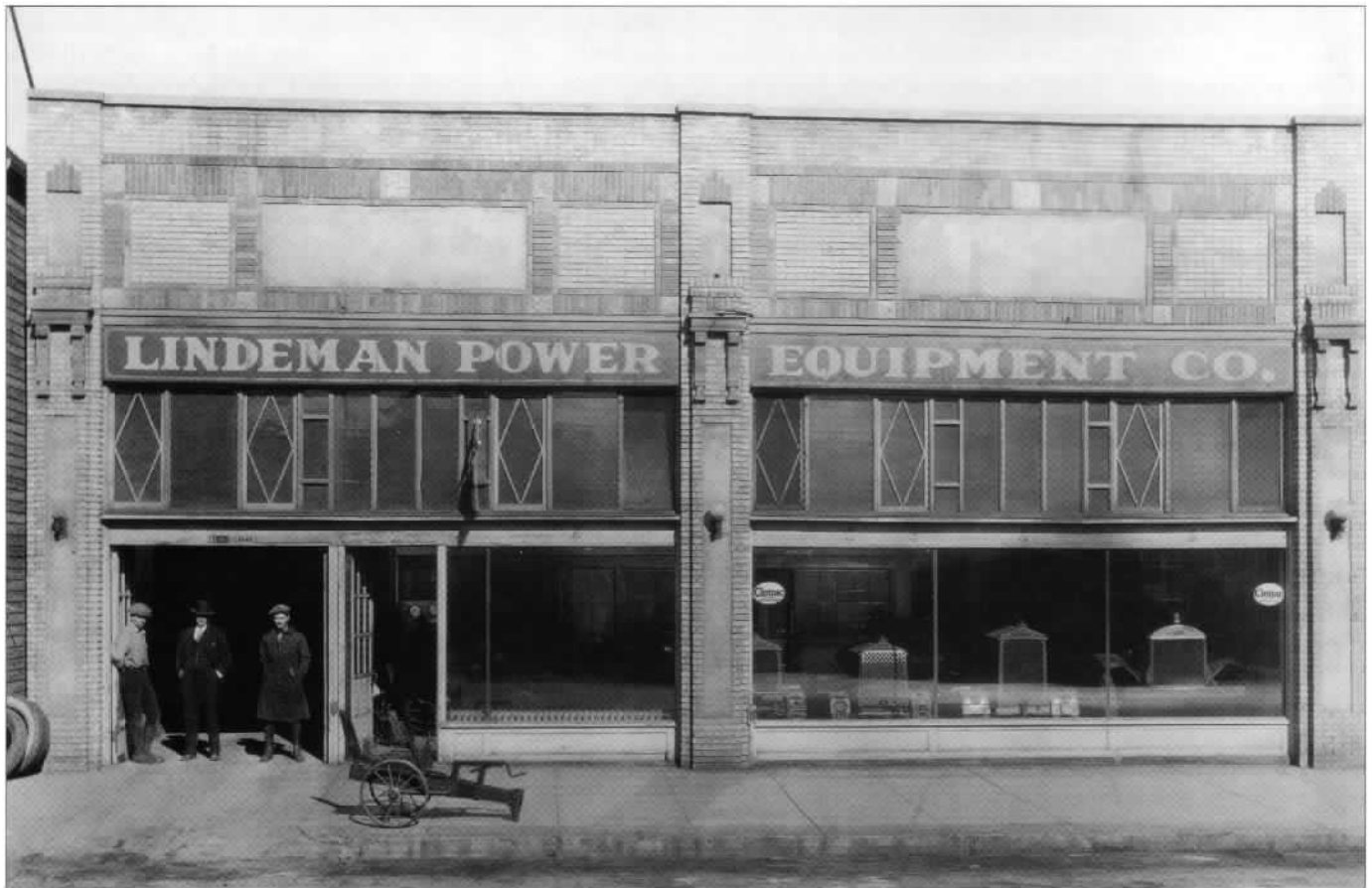
The store front (formerly a Cadillac dealership) of the Lindeman Power Equipment Company in 1927. The firm became dealers for the "Cletrac" line of crawler tractors in 1926. by 1928, the Lindeman Power Equipment Company would also become John Deere dealers, and the Lindeman brothers' experience with crawler tractors would lead them in a new direction. The gent on the left in the doorway is none other than Jesse Lindeman, rightfully credited with being the lead designer and visionary of the family.
