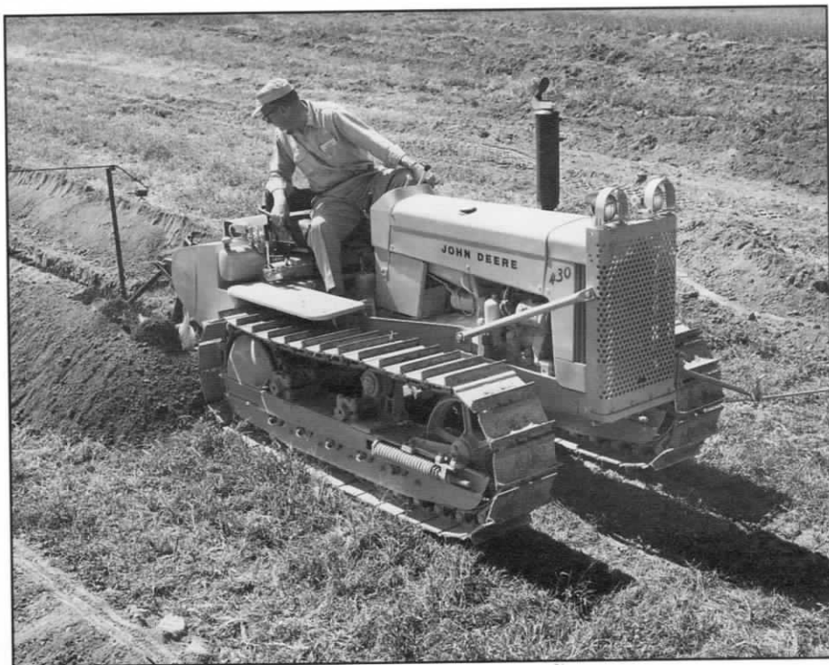
A 430 five roller crawler in industrial yellow paint, equipped with Auburn trencher, September 1958.
