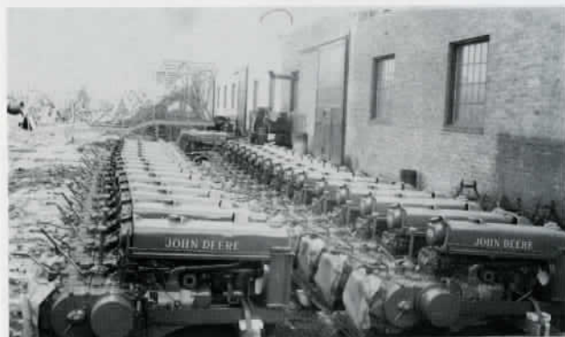
Shipment of "BO" tractors, without wheel equipment, from the John Deere Waterloo Tractor Works.
